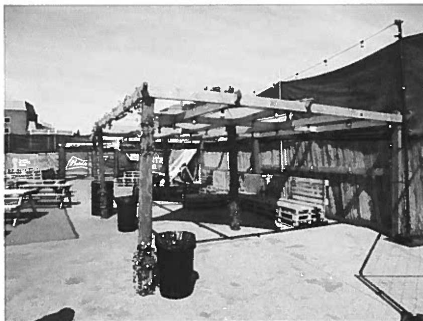
One of the wooden structures at Station Hill
